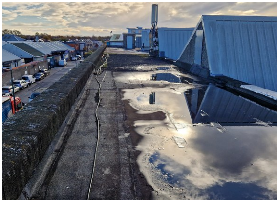
The existing concrete and asphalt roof prior to preparation.
