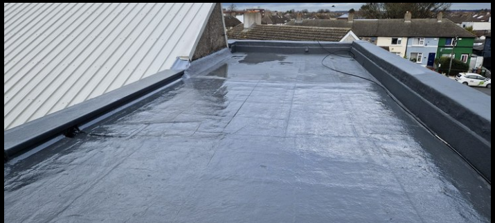
The completed TriRoof FLEX overlay across the deck, upstands and parapet.
