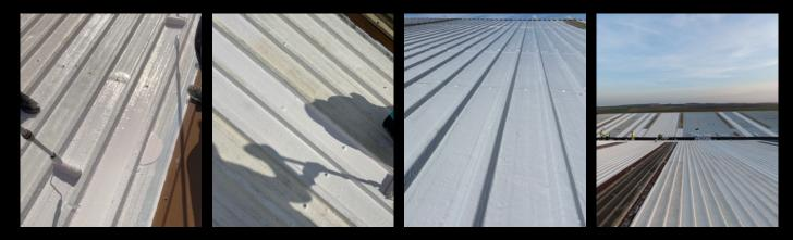
The project officially commenced in early February, with on-site installation of the large-scale commercial flat roof beginning in March. Despite the technical complexity of applying the HPX system over corrugated sheeting—and the added requirement for additional primer due to substrate conditions—the ECMS team successfully completed the 6,000 m² roof by March 31st, comfortably within the seven-week schedule.
